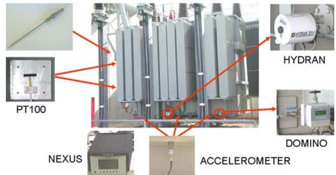
Fig. 2. Placement of sensors in the monitored power transformers
